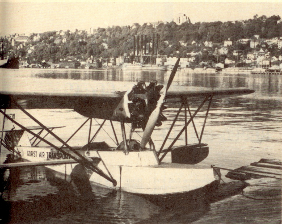
An Eastman E-2 Sea Rover flying boat of Gorst Air transport, photographed on Lake Union in the heart of Seattle, Wash. Note the open cockpits and rudimentary lower wing. Photo by Gordon S. Williams.
